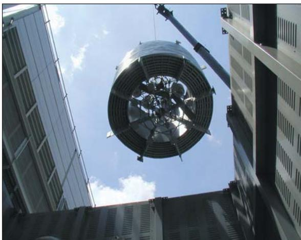
*A crane lowered the six five-ton reactor coils into place. Each reactor is a stack of three coils rated at 2000 amps each.*
