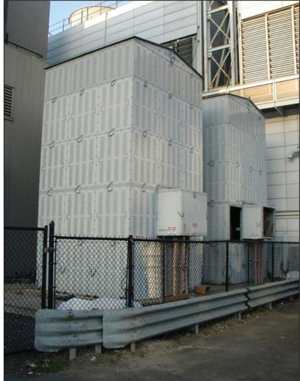
*The new reactors stand side by side at the edge of the campus. Because the new units are taller than the lower-capacity reactors they replaced, the roofs were raised and another cubicle section was added at the top of each enclosure.*
