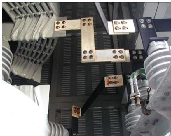
*Phoenix Electric also manufactured the internal copper buswork for the two reactors. Each reactor is wired separately to the university's generator bus, providing redundancy.*
