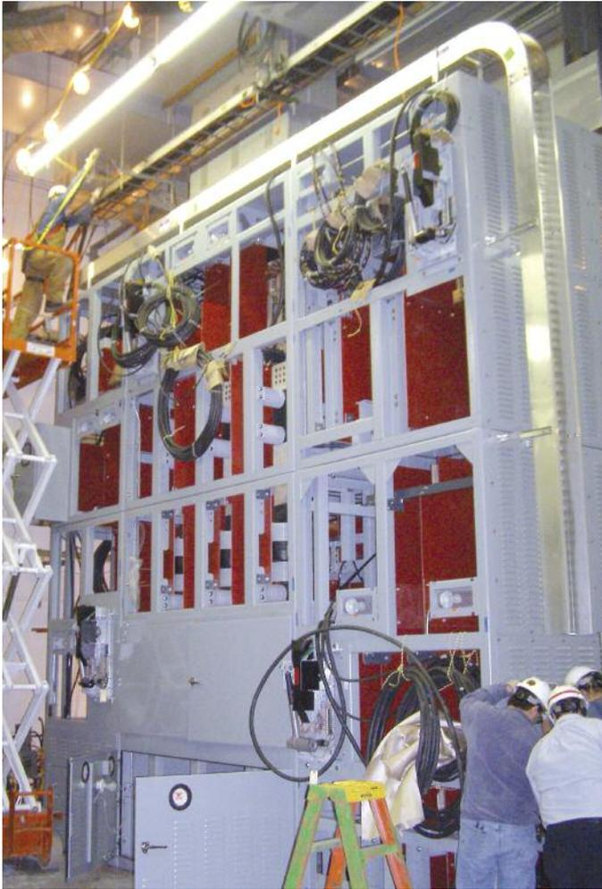
**Above: Designed and built by Phoenix Electric Corporation for one of the Muddy Run facility's eight generators, this six-cubicle switchgear/circuit-breaker unit stands approximately 5.6m high and weighs about 15 tons**
