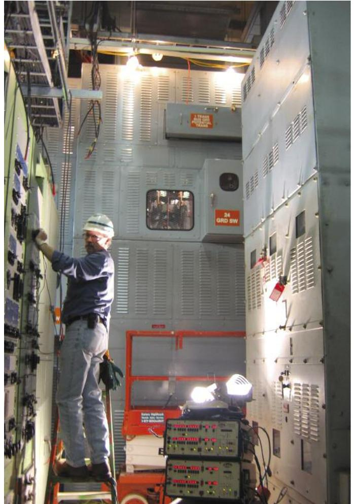
**Inside the Muddy Run pumped storage facility in southeastern Pennsylvania, a technician checks newly installed Phoenix Electric switchgear prior to commissioning**
